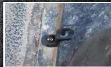
Figure 8 - Proper Hook Orientation
