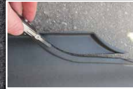
Figure 10 - Trimming Along Rib
