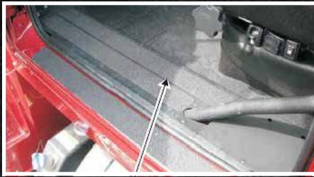
Figure 4 - Driver Side Electrical Tray
